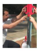
**Step 9 -** Using a 6" heavy-duty safety film squeegee, wipe from the center with firm downward and outward movements, removing water and air bubbles trapped between the film and the glass.
