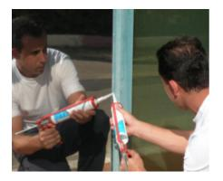
**Step 14 - Edge Sealing:** Allow film to dry for 24 hours, then within 72 hours, complete by edge sealing on all four edges.
