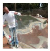
**Step 7 -** Remove release liner from film and spray the exposed adhesive layer with plenty of wetting solution.
