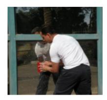
**Step 8 -** Position the film on the window with wet adhesive side on the glass.
