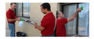
**Step 7 alternative -** Separate release liner from the precut film (rolled with liner outside) and spray the exposed adhesive layer generously with wetting solution. Make sure to wet the window with plenty of wetting solution!
