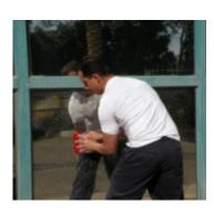
**Step 12-** Wet the film surface again, and pressing hard with the squeegee, wipe out from the center until all the air bubbles and remaining water has been removed from the edges.
