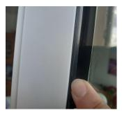
Start at the edge of the window. Remove the liner with one hand and attach the edge sealing tape with the other hand partly onto the window film and partly onto the glass pane for a good sealing result.
