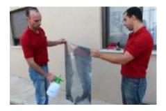
**Step 2:** Spray film on both sides to avoid static (less dirt in installation) and flatten the film.
