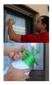
**Recommended Tools:** Spray bottle with wetting solution (liter tap water and 4 drops of detergent-free soap); Scraper; Cutter knife; 6" heavy-duty safety film squeegee; Paper towels.
