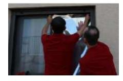
**Step 7:** Position the film on the window with wet adhesive side on the glass.
