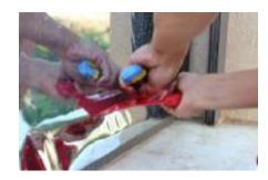
**Step 9:** Trim the edges of the film adjacent to the window frame, using the Stanley knife and the Edge Tool.
