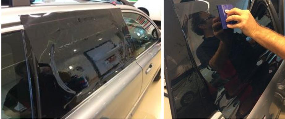
As next step, shrink the film to the window shape, heating the film with a heat gun. When heat shrinking the film, pay attention to heat the film uniformly and do not hold the heat gun too close to the surface to avoid local overheating.
