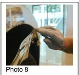
• Keep the squeegee edge wet during the entire application process, paying attention to rewet the squeegee upon final re-squeegeeing of all edges, and the entire graphic to ensure secure adhesion to the substrate. As shown in photo 9.
