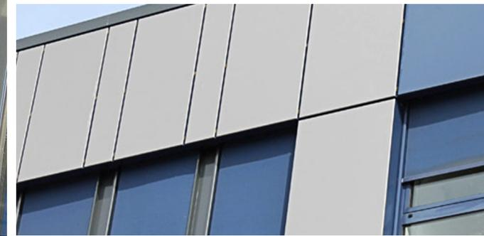
“ 2500 m<sup>2</sup> of Facade Film were used during the project, applied to window frames, window sills, attic components and metal facade sections. Project duration was three months, with three applicators.
