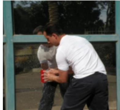
**Step 8** - Position the film on the window with wet adhesive side on the glass.
