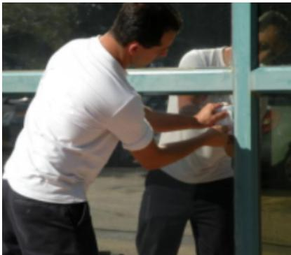
**Step 12**- Wet the film surface again, and pressing hard with the squeegee, wipe out from the center until all the air bubbles and remaining water has been removed from the edges.
